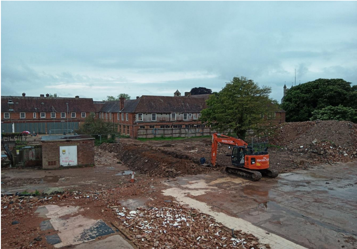
Plate 1: Looking south west at the site from north east corner
